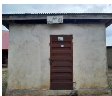
Exterior view of the food store showing concrete walls, corrugated sheet roofs and lockable doors
